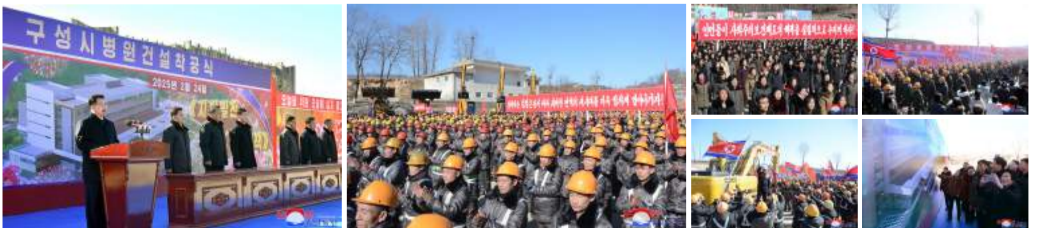
The construction of the Kusong City Hospital starts with due ceremony on February 24.
